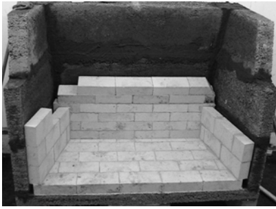
Figure 8. Firebrick Installation
