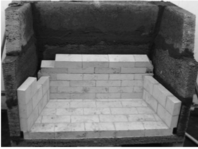
Figure 9. Firebrick Installation
