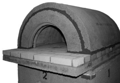
Figure E Assembled Oven With Extension, Prior to Chimney Installation
