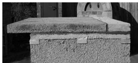
Figure E Assembled Oven With Extension, Prior to Chimney Installation
