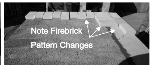
Figure E Assembled Oven With Extension, Prior to Chimney Installation
