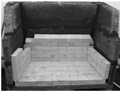
Figure 9. Firebrick Installation
