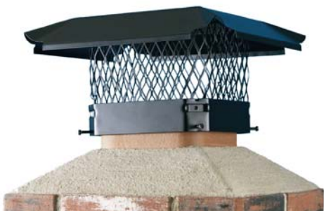
Figure 15. Mortar Cap and Chimney Cap
