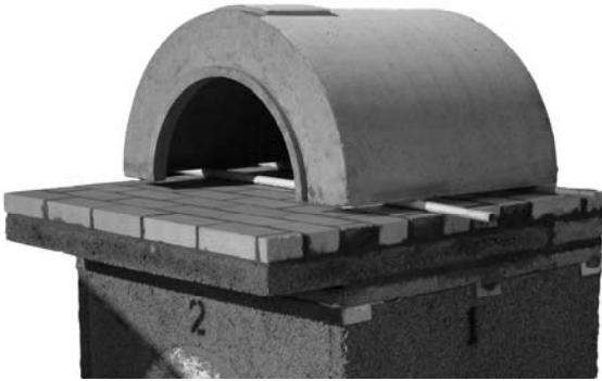
Figure C Use shims or other temporary spacers during mortar application
