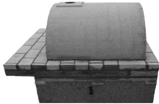
Figure D Liner Shell installed
