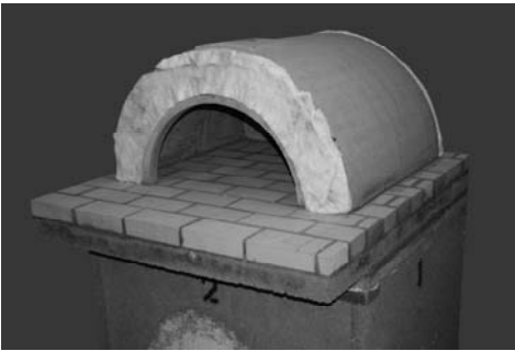
Figure G Cut blanket to fit front wall
