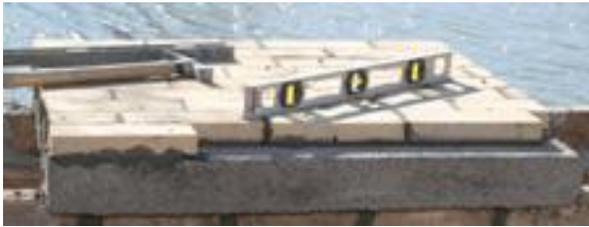
Figure 4. Install Firebrick on Baseplate
