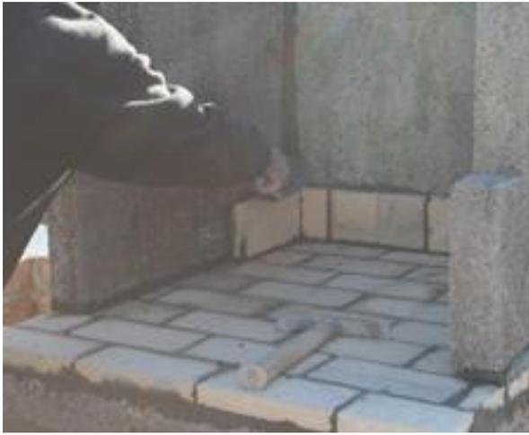
**Figure 7. Line Box with Brick**
