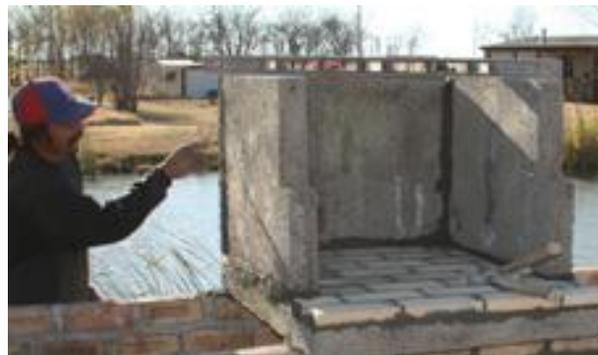
Figure 6. Set Side Walls and Back Plate
