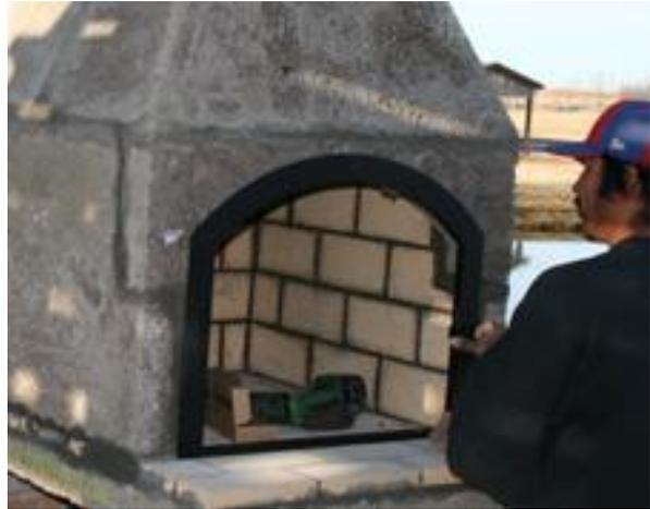
**Figure 9. Install Frame and Door**
